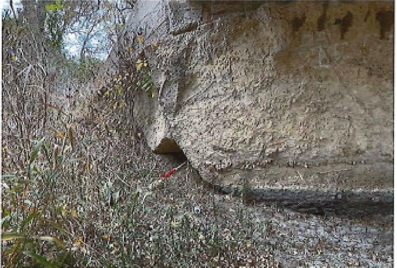
UNDERMINED EAST CORNER WINGWALL LOOKING NORTHEAST
