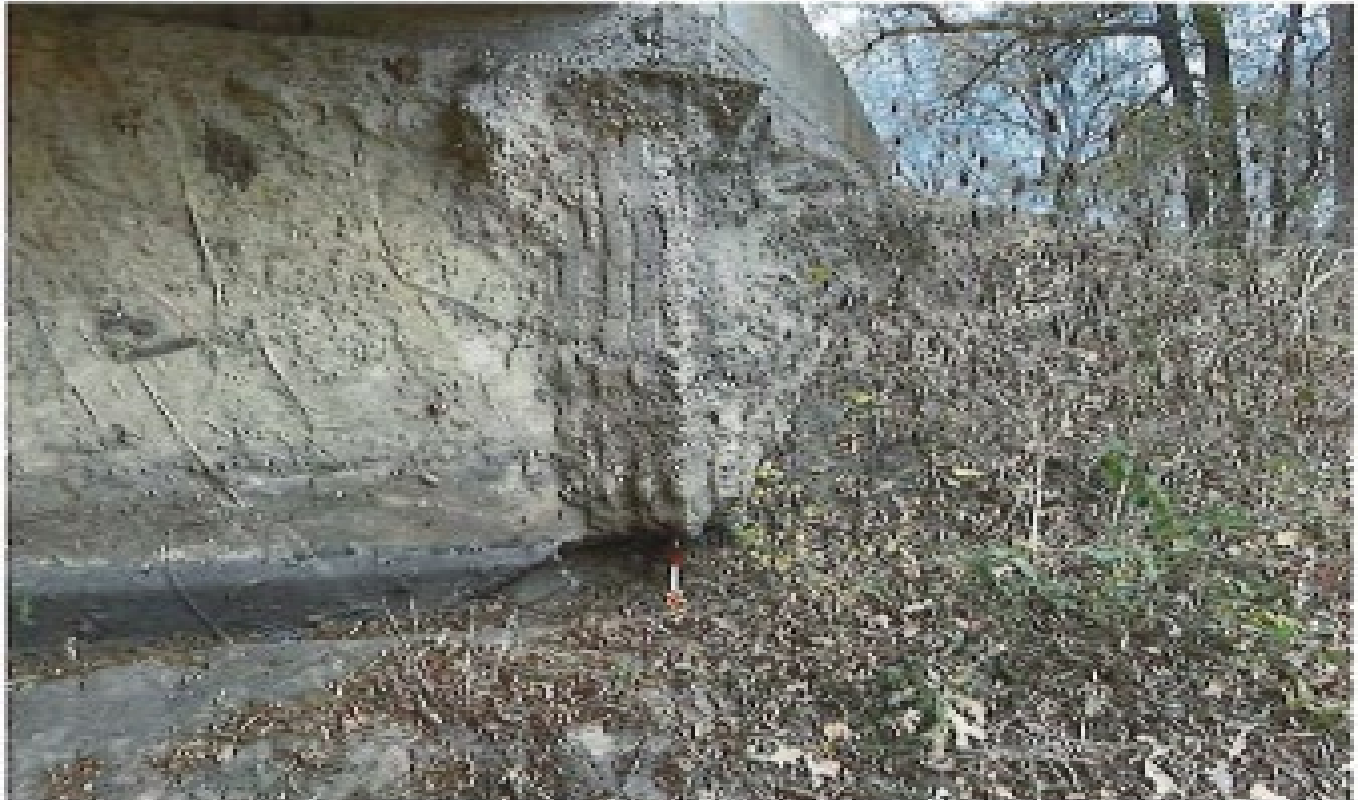
UNDERMINED EAST CORNER WINGWALL LOOKING NORTHEAST
